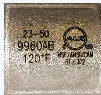
Design Temperature Listed On Valve Body
